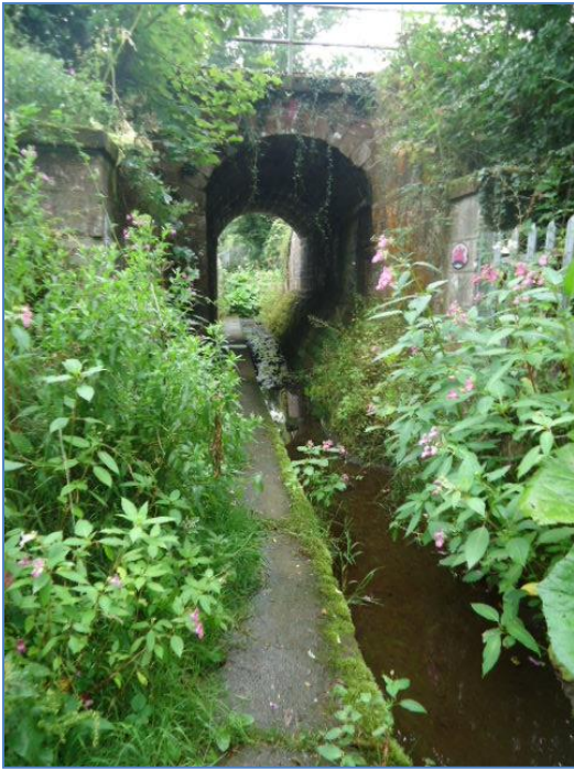
Gully under the railway
